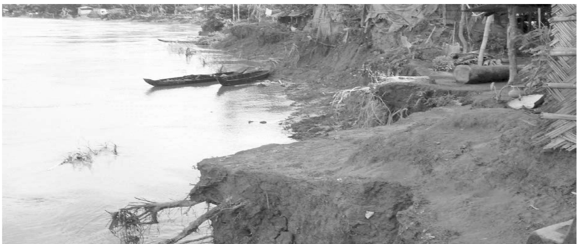
Figure 2: River bank erosion
